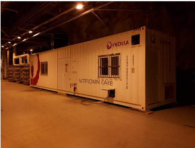
Figure 1. The containerised Actiflo® Mini Carb piloting system within Viikinmäki WWTP.
